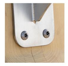
Stainless steel screws and/or screws covered with plastic caps,
