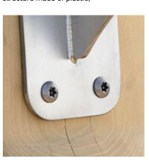
Stainless steel screws and/or screws covered with plastic caps,
